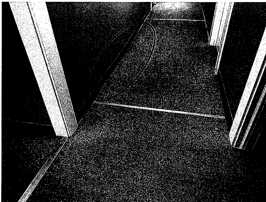
Photo #1 – Third-floor hallway movement
